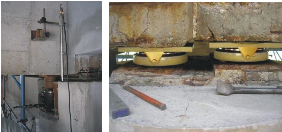
Fig 15 Unit for lifting with hydraulic jackets and new bearings
