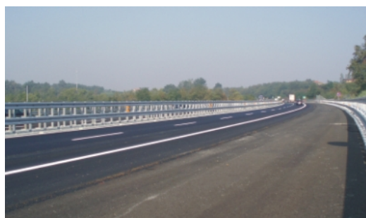
Fig. 20 Road view of new Solbrito viaduct
