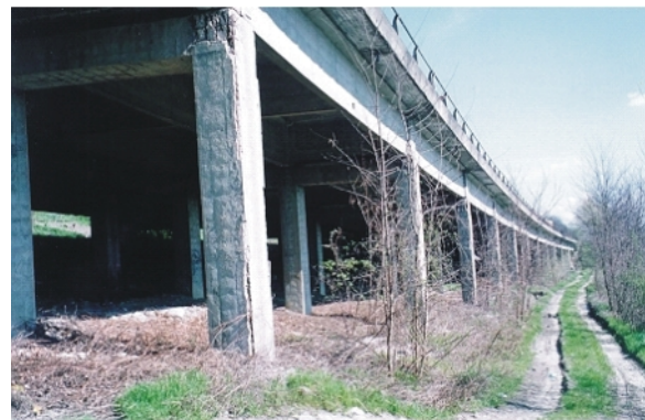
Fig. 4 Lateral view of bridge
