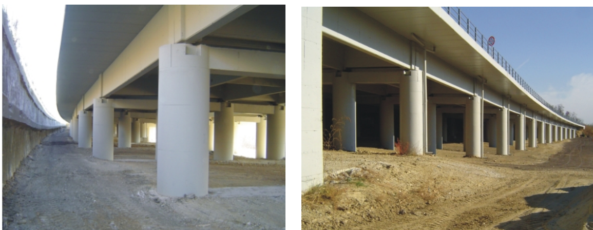
Fig. 19 Panoramic views of Solbrito viaduct after rehab
