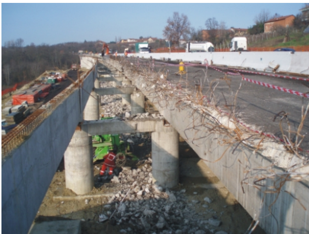
Fig. 11 Preparing works for the new slab
