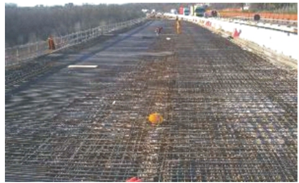
Fig. 12 Steel bars casting and connectors
