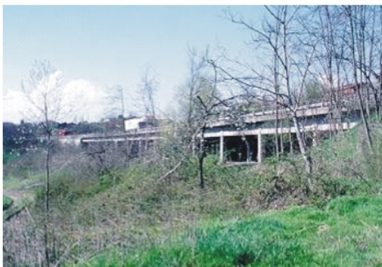
Fig. 3 Panoramic views of bridge
