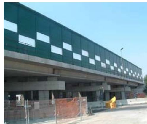
Opera 22 - Posa Trevi in c.a.p.
