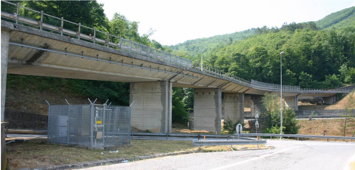
Fig. 1. View of the "Carrodano" viaduct (neighbouring the Levanto town, Liguria, Italy)
