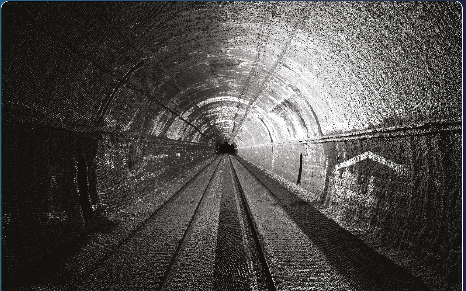
3D Point Cloud: Bologna-Florence Railroad; Inside of the Gabbolana Tunnel
